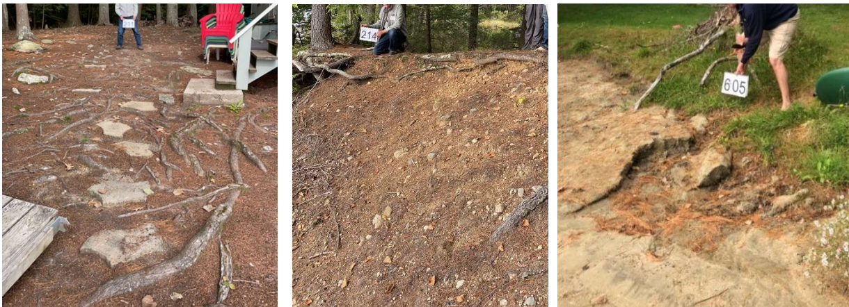
Surface erosion on a pathway leading to the lake exposes tree roots and bare soil (site 2-11, left). Shoreline bank erosion delivers sediment directly to the lake (site 2-14, center). Runoff from developed areas causes gully erosion on a Pocasset Lake shorefront (site 6-05, right).
