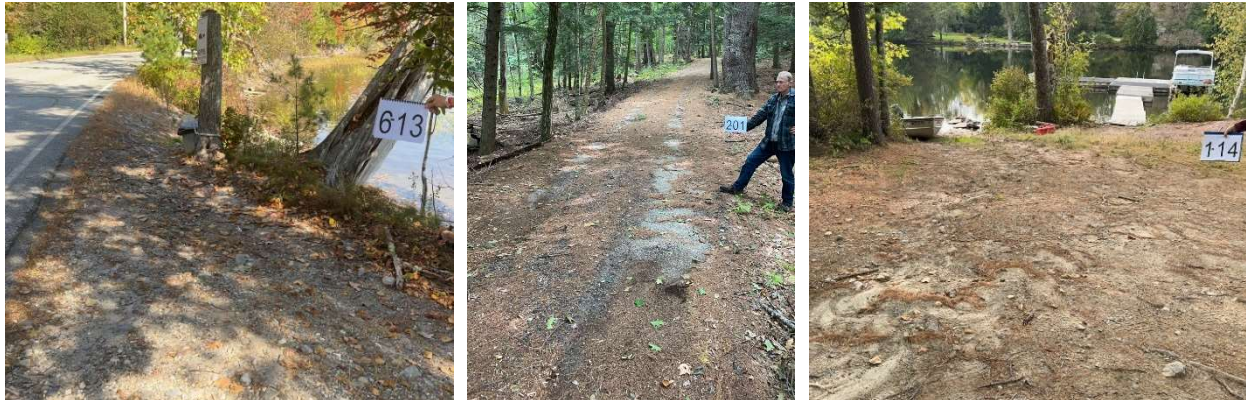
Road shoulder and surface erosion on a town road at the carry-in launch location on Pond Road (site 6-13, left). Road surface erosion on a private gravel camp road (site 2-01, center). Runoff exiting a driveway causes rill and gully erosion and delivers pollutants directly to the lake via boat and dock access points (site 1-14, right).
