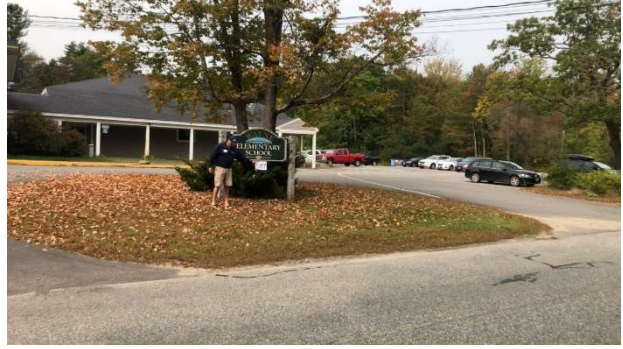
Medium impact erosion site 6-07 has large areas of impervious surfaces that deliver surface runoff across Pond Road toward Pocasset Lake.
