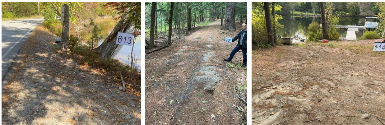
Road shoulder and surface erosion on a town road at the carry-in launch location on Pond Road (site 6-13, left). Road surface erosion on a private gravel camp road (site 2-01, center). Runoff exiting a driveway causes rill and gully erosion and delivers pollutants directly to the lake via boat and dock access points (site 1-14, right).
