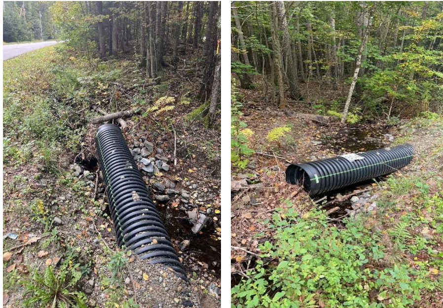
High impact erosion site 3-04 on N. Wayne Road in North Wayne. Snowmobile trail cross-culvert failure.
