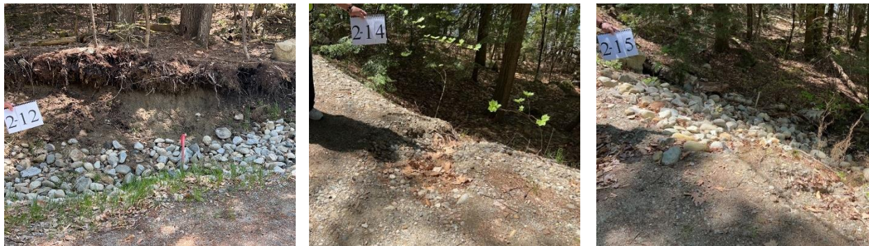
Private road sites 2-12, 2-14, and 2-15 documented on Holman Terrace in Sector 2.
