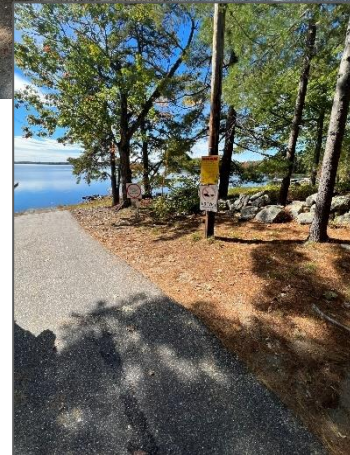
Erosion at roof driplines and adjacent common spaces (top) and boat launch (bottom) documented at site 9-14 in Wayne
