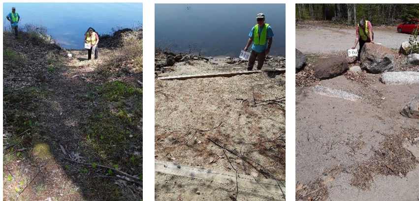
Example sites identified in the Stinchfield Beach neighborhood in Sector 7: Site 7-06 (left) erosion on a shorefront pathway, site 7-11 (middle) unstable soils on a steep slope, and site 7-09 (right) runoff from a town parking lot is creating a channel with flow to Androscoggin Lake.
