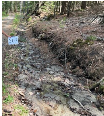
Erosion sites identified on Dole's Beach Road / The Boulevard in Sector 2. Runoff over-topping the road (Site 2-06) and eroding a channel in the road surface, and overwhelmed ditch full of sediment that drains to Androscoggin Lake (Site 2-03), and an unstable culvert outlet (Site 2-09).
