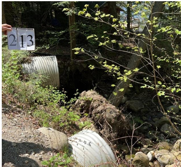
Bank failure at a culvert outlet (site 2-13) on Holman Terrace in Sector 2.
