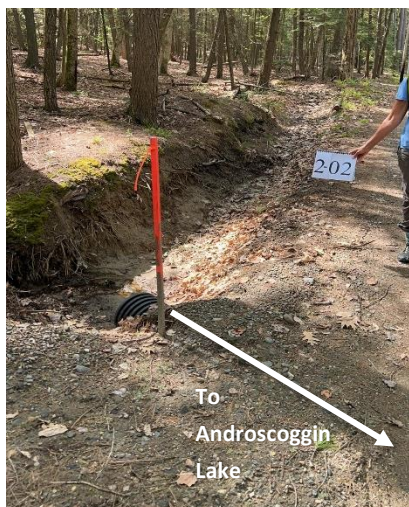
Ditch, culvert, and road surface erosion identified on a private gravel road that drains to Androscoggin Lake.
