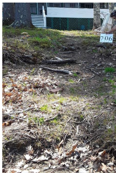
Surface erosion on a pathway leading to Androscoggin Lake.
