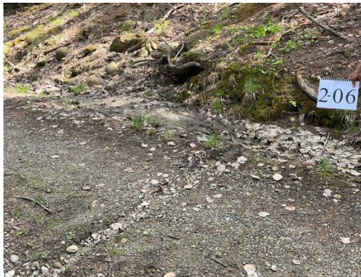
Erosion sites identified on Dole's Beach Road / The Boulevard in Sector 2. Runoff over-topping the road (Site 2-06) and eroding a channel in the road surface, and overwhelmed ditch full of sediment that drains to Androscoggin Lake (Site 2-03), and an unstable culvert outlet (Site 2-09).
