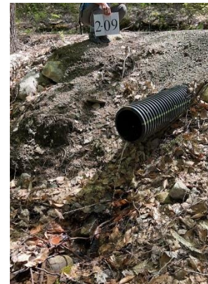
Erosion sites identified on Dole's Beach Road / The Boulevard in Sector 2. Runoff over-topping the road (Site 2-06) and eroding a channel in the road surface, and overwhelmed ditch full of sediment that drains to Androscoggin Lake (Site 2-03), and an unstable culvert outlet (Site 2-09).
